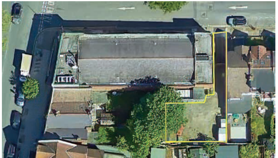
Spare land: An aerial view shows the car park area at the rear of the Phoenix Cinema
