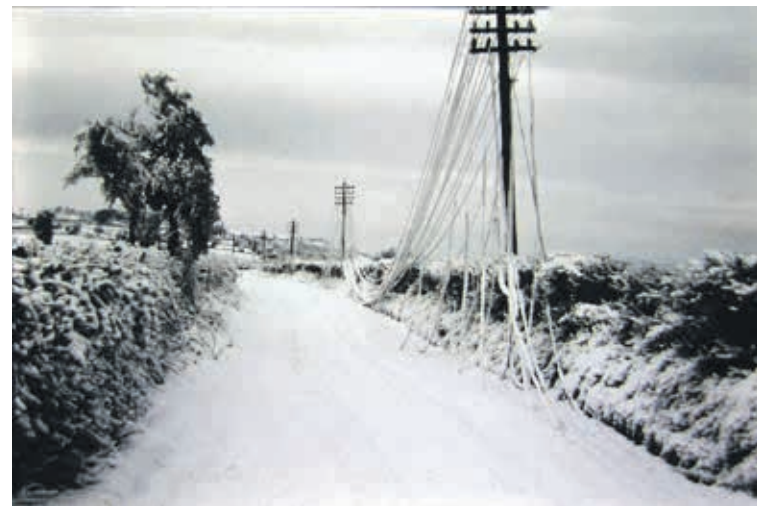
The weight of snow and ice stretched the copper telephone wires until they reached the ground. East Dundry Lane, Somerset, January 1963
