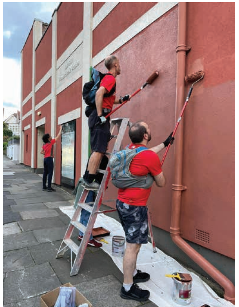
... and repaint the side of the Phoenix Cinema.
