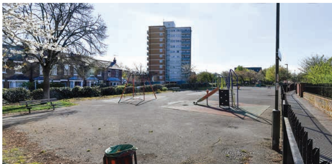
Redesign: The playground in Market Place is in line for a revamp. Photo Mike Coles
