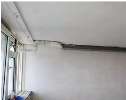
Outlet: The ducting ends at one of the flat's windows
