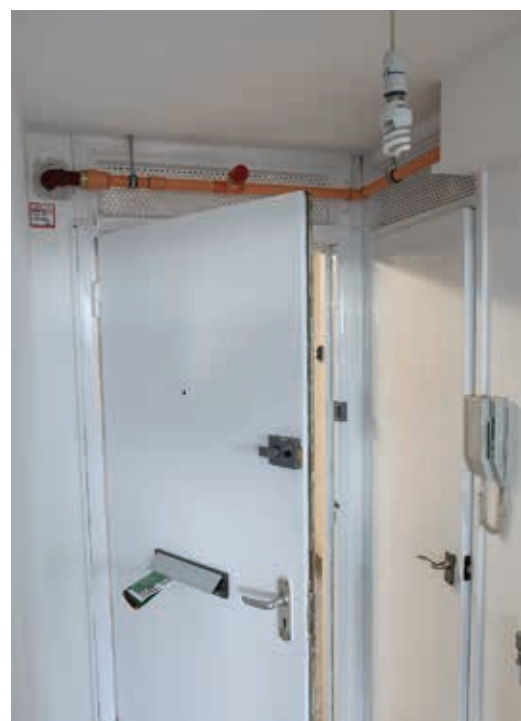
Work in progress on the new sprinkler system being installed at Prospect Ring. Photo Mike Coles
