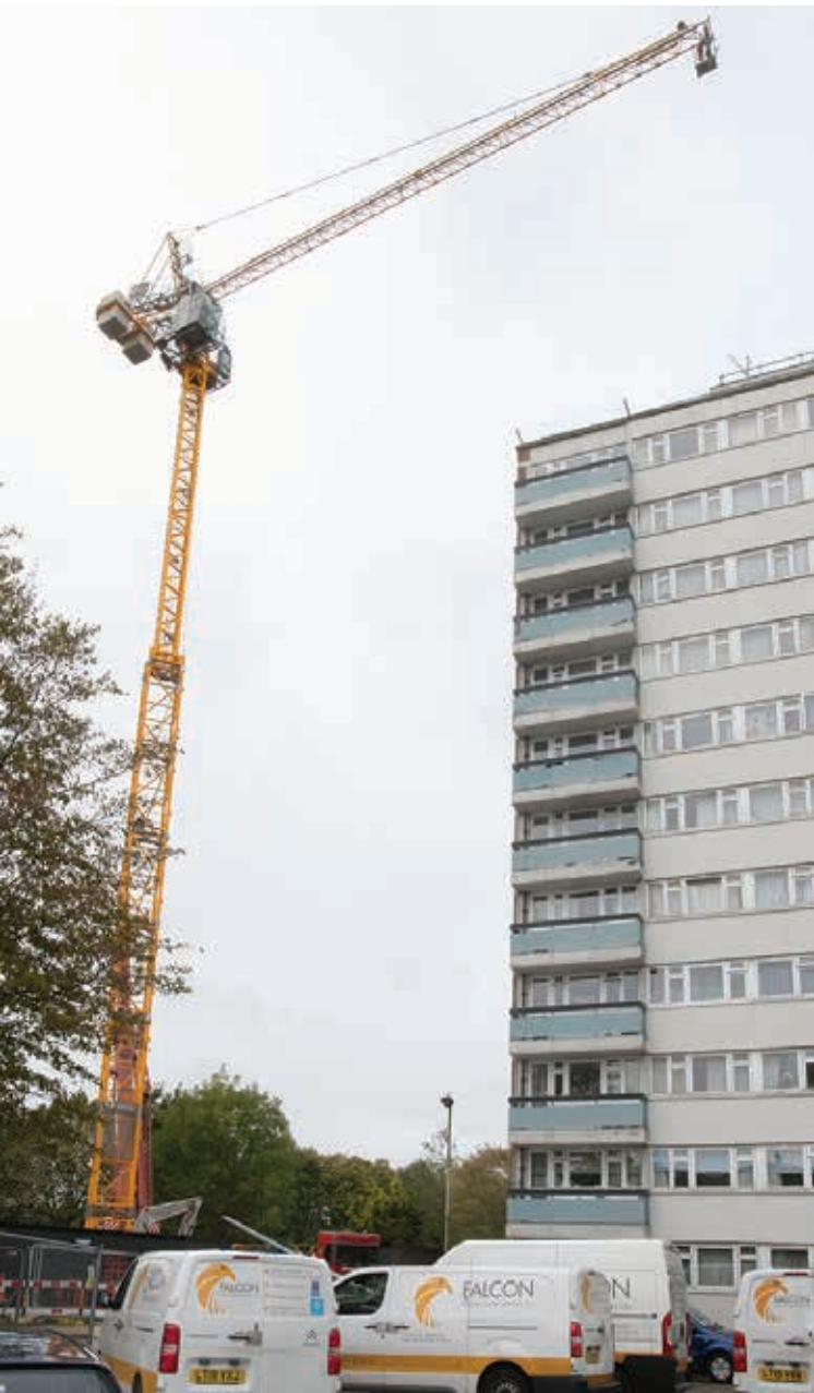
The tower crane is erected at Prospect Ring for the new block. Photo Mike Coles
