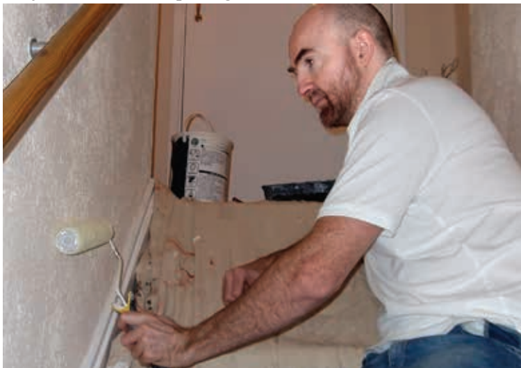
Lick of paint: Michael Dudman at work.
