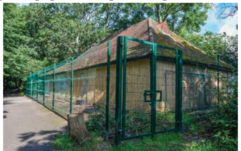
The pavilion, after it was made safe two years ago.
