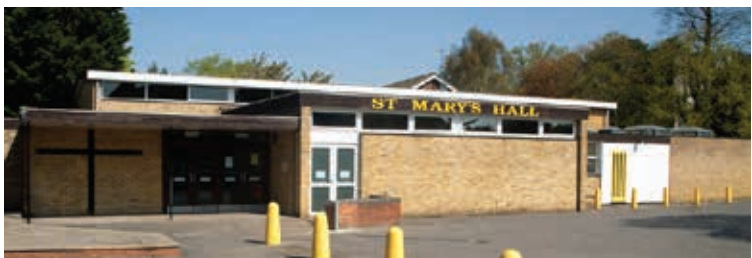
Finchley Central: St Mary-at-Finchley Social Centre, 1958, by Kenneth Wood; post-war church social centre, designed by Kenneth Wood, better known for his house designs in South London and Surrey.
