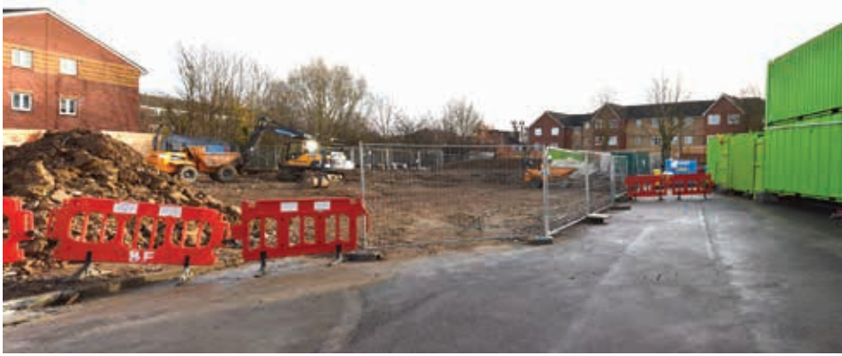
The Old Barn building site in November. Photo Mike Coles
