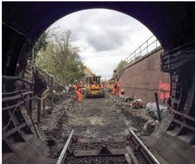
Tunnel vision: Contractors re-lay the Northern line track at East Finchley. Photo courtesy ???
