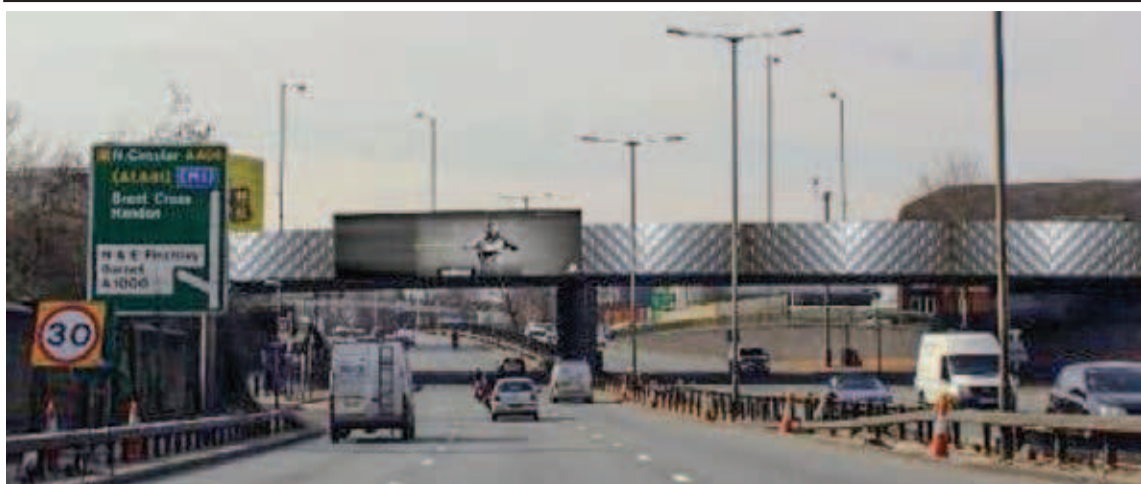
Heads up: How the advertising screen will look will look to westbound drivers on the North Circular, taken from the council's planning statement
