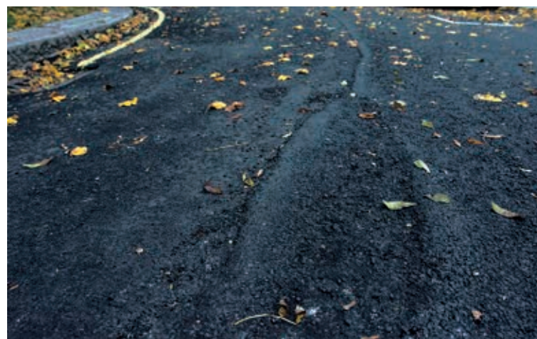
Some of the resurfacing work in Abbots Gardens Photo Mike Coles
