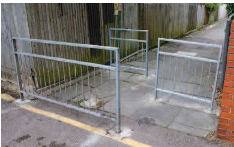
Badly repaired: The motorbike barriers between Durham Road and Creighton Avenue'
