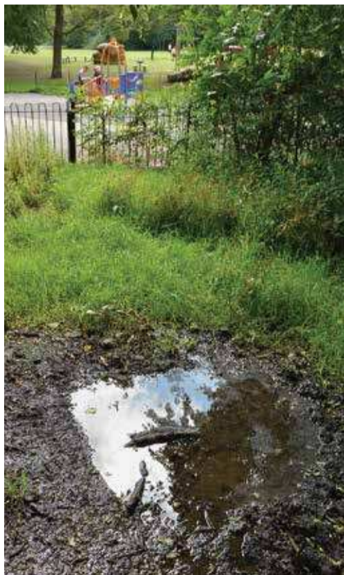
A large puddle of still water from a leak near the children's playground in Cherry Tree Wood. Photo Mike Coles
