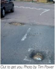
formation of potholes as water expands when it freezes to form ice. Barnet Council has had to repair more than 9,000 potholes
