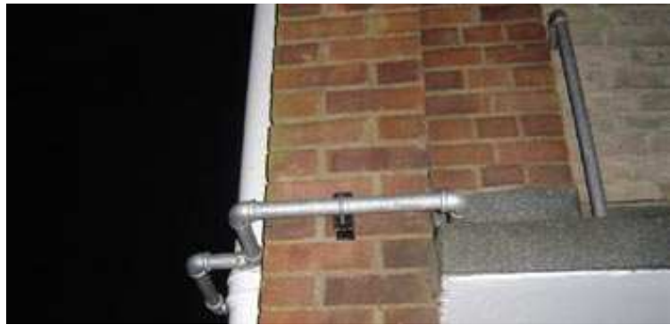
The new gas pipes attached to homes in Park Farm Close. Photo by Melanie Bruck
