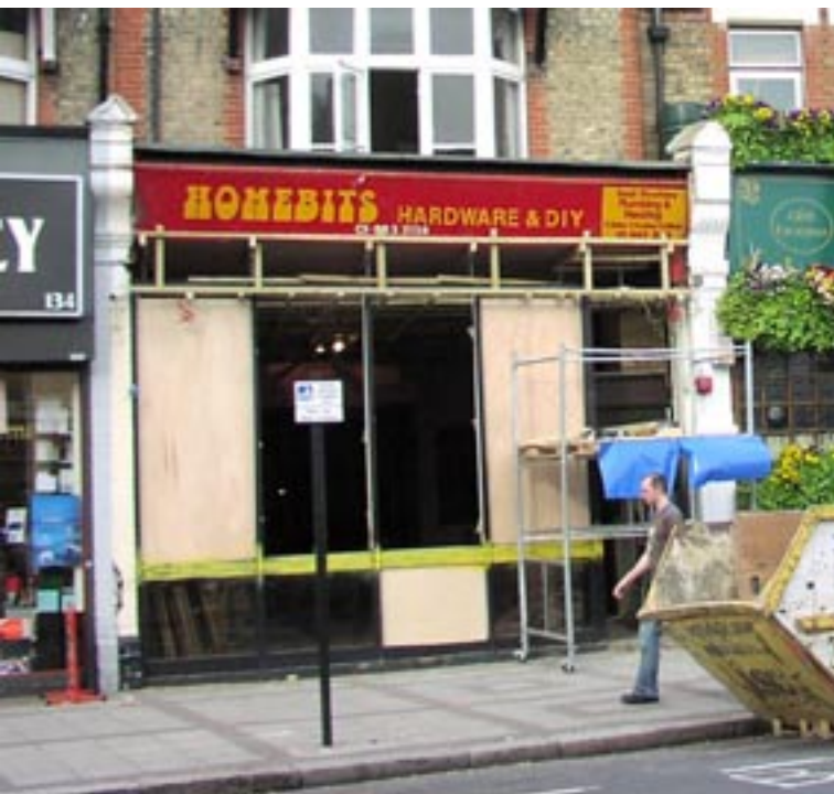
The refurbishment of the restaurant next to Madden's has exposed the old shop sign - who remembers Homebits and when did it close? Picture by Diana Cormack
